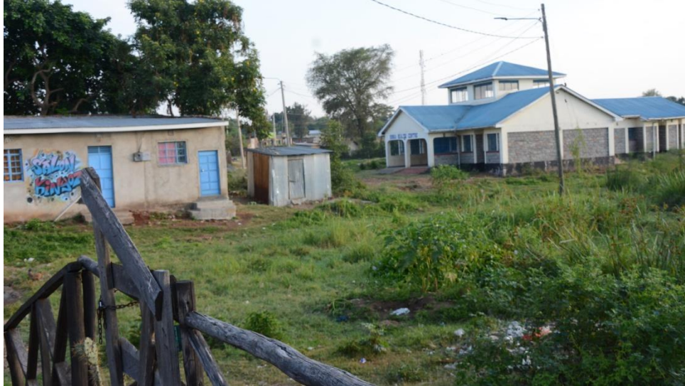
Figure 1: A church and Business Premises Encroaching in Dunga Wetland
