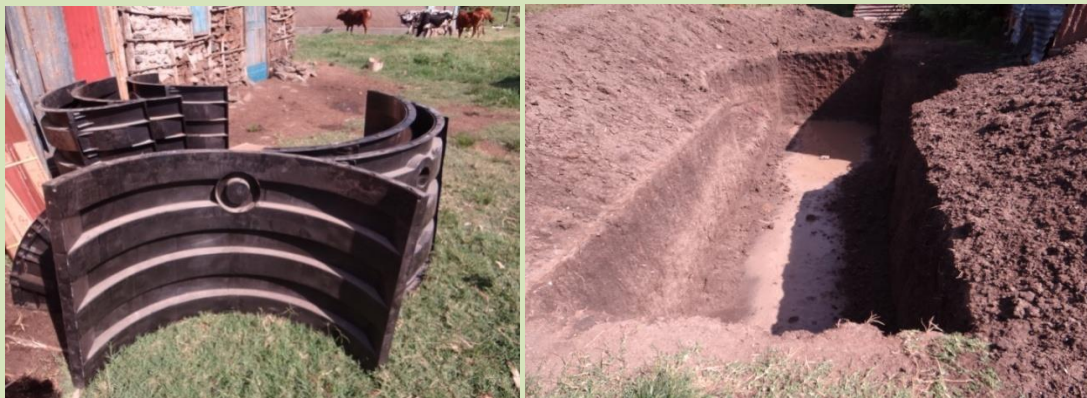
Photo 9: Materials and Excavation for a Simgas Biogas Digester
